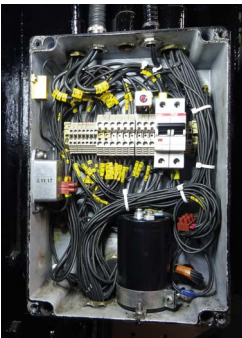
Above centre: Inside ADA connection box with wiring and over-voltage crowbar in place on the left.
