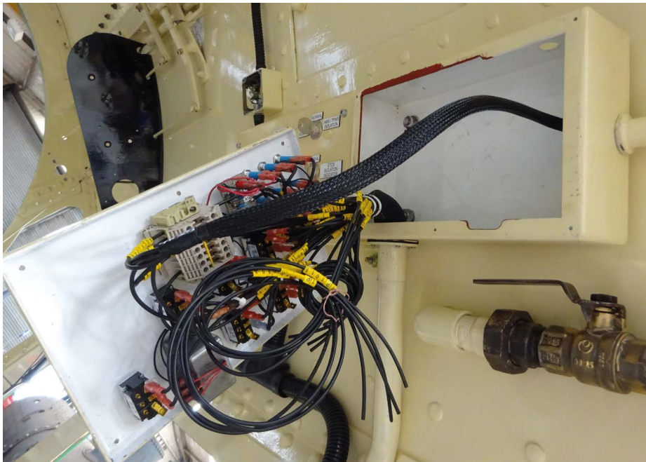
AS Control Panel during final wiring.
