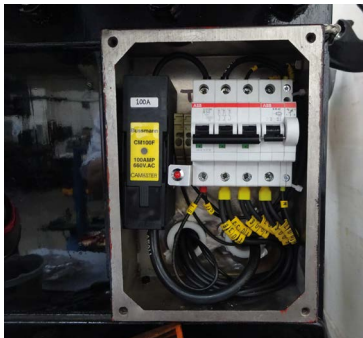
Outside ADA connection box with all components and wiring in place.
