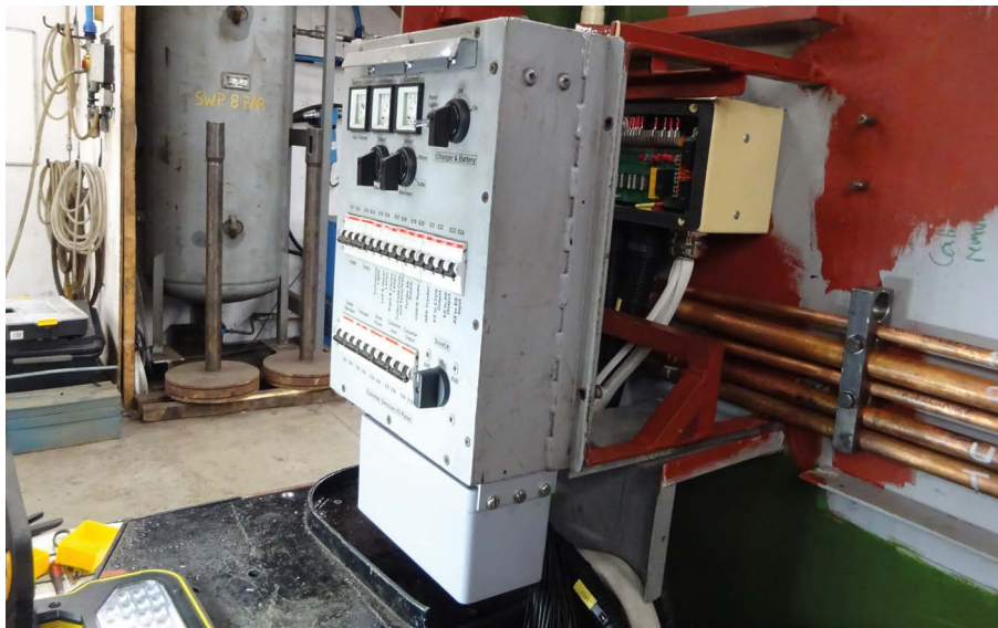
Right: ES I/O Panel in place with new wiring box underneath.
